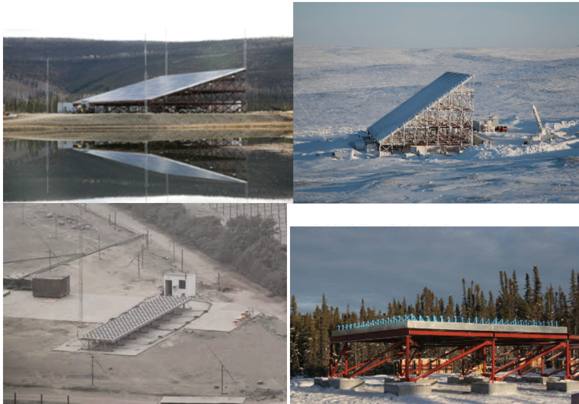
Figure 2.1 (Top Left) The Poker Flat Incoherent Scatter Radar (PFISR) 128-panel AMISR system. (Top Right) The Resolute Bay Incoherent Scatter Radar (RISR-N) 121-panel AMISR system. (Bottom Left) The 14-panel AMISR system at the Jicamarca Radio Observatory in Peru. (Bottom Right) The 16-panel AMISR system at the High Altitude Auroral Research Program (HAARP).
