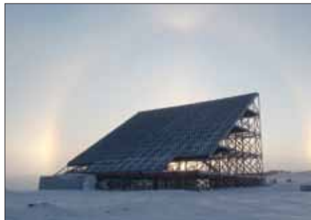
1 (Left): North face of the Resolute Bay Incoherent Scatter Radar (RISR-N), which probes the plasma parameters in the polar cap ionosphere, and (right) crossed dipole antennas on RISR-N. (C Heinselmann)
